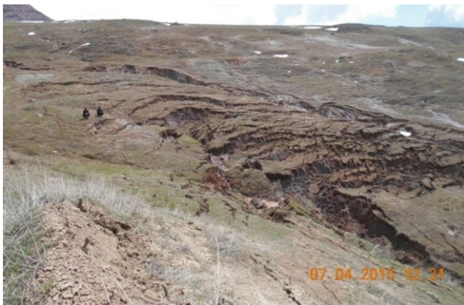
Fig. 5 Transverse cracks in the area of formation of the landslide Khandiza
