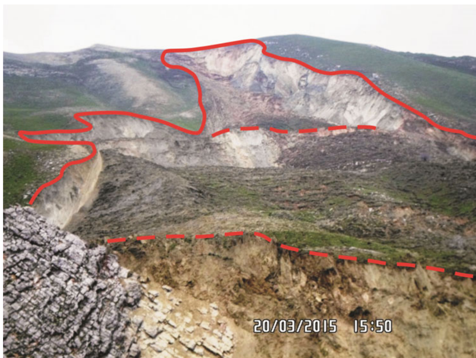
Fig. 1 General view of Chaigul landslide
