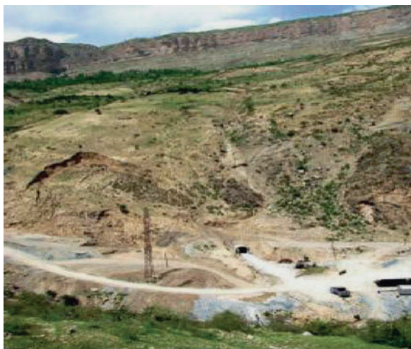
Fig. 17.6 Khandiza block landslide site
