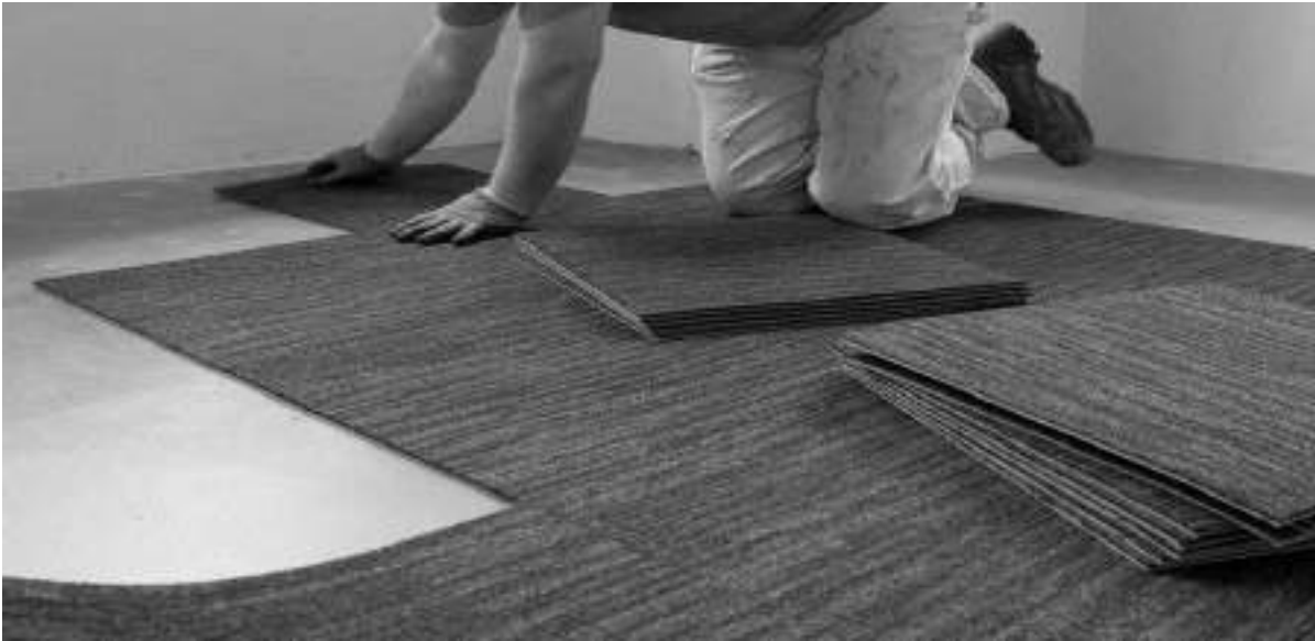
Figure 3 CARPET TILE INSTALLATIO
